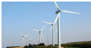
Wind Power Generation
